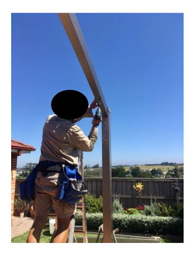
It may be an idea to not fully tighten the bolts until the end. A 1mm or 2mm 'wiggle' on a slightly loose bolts might be helpful – But remember to fully tighten at the end of the job if you do this!
